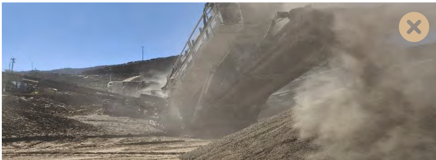
Dust generated from crushing activities is one of the major sources of airborne pollution. An example of ineffectively controlling dust at the crusher.
